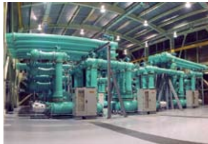
ABB gas-insulated switchgear.
