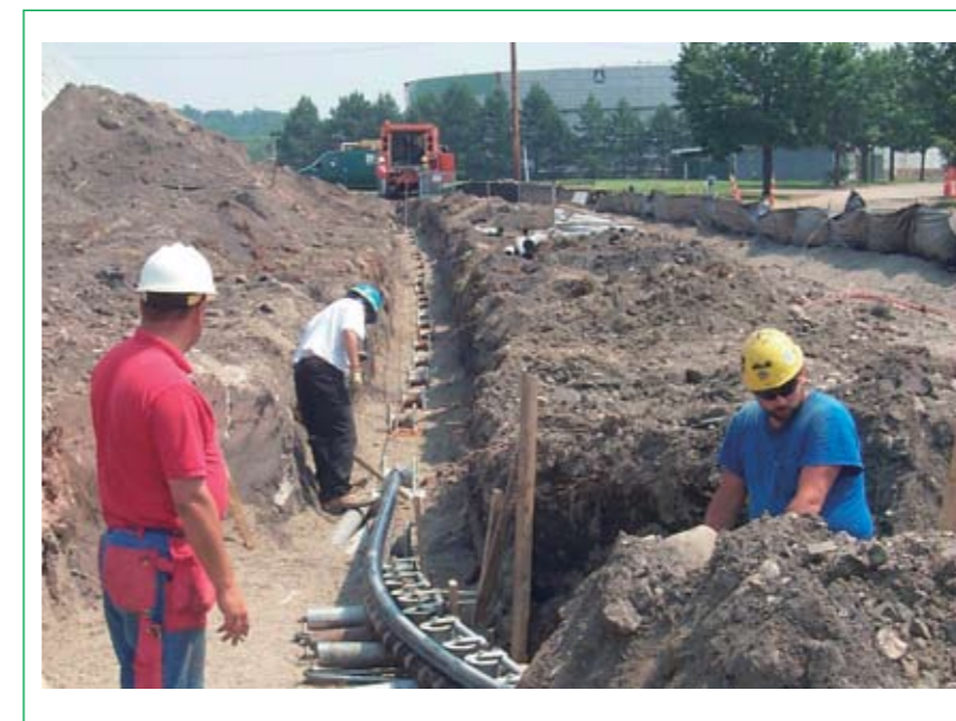
Figure 4: HVDC Light cable laying with minimum environmental intrusion.
