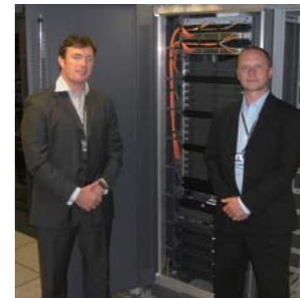
Andrew Clarke and William Barrell, Infrastructure Project manager, pictured with Chloride's Active UPS. Deployed across ten communications rooms to support the IPT deployment, Chloride's Active 3000VA is installed in standard cabinets with MODBUS and SNMP cards, to ensure that voice communications are not lost in the event of power failures. Testing showed that the Chloride batteries will support the system at full load for 30% longer than the designed specification.
