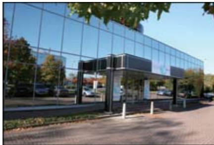
Dialog's impressive 1400m 2 new facility in Swindon, UK is the new home for 85 employees with space for expected expansion to 125.
